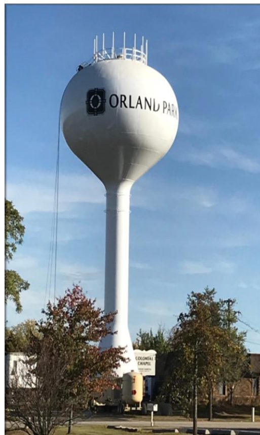
Exterior Painting & Modernization Concept
