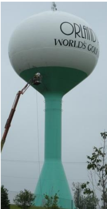
Existing Condition of Water Tower
